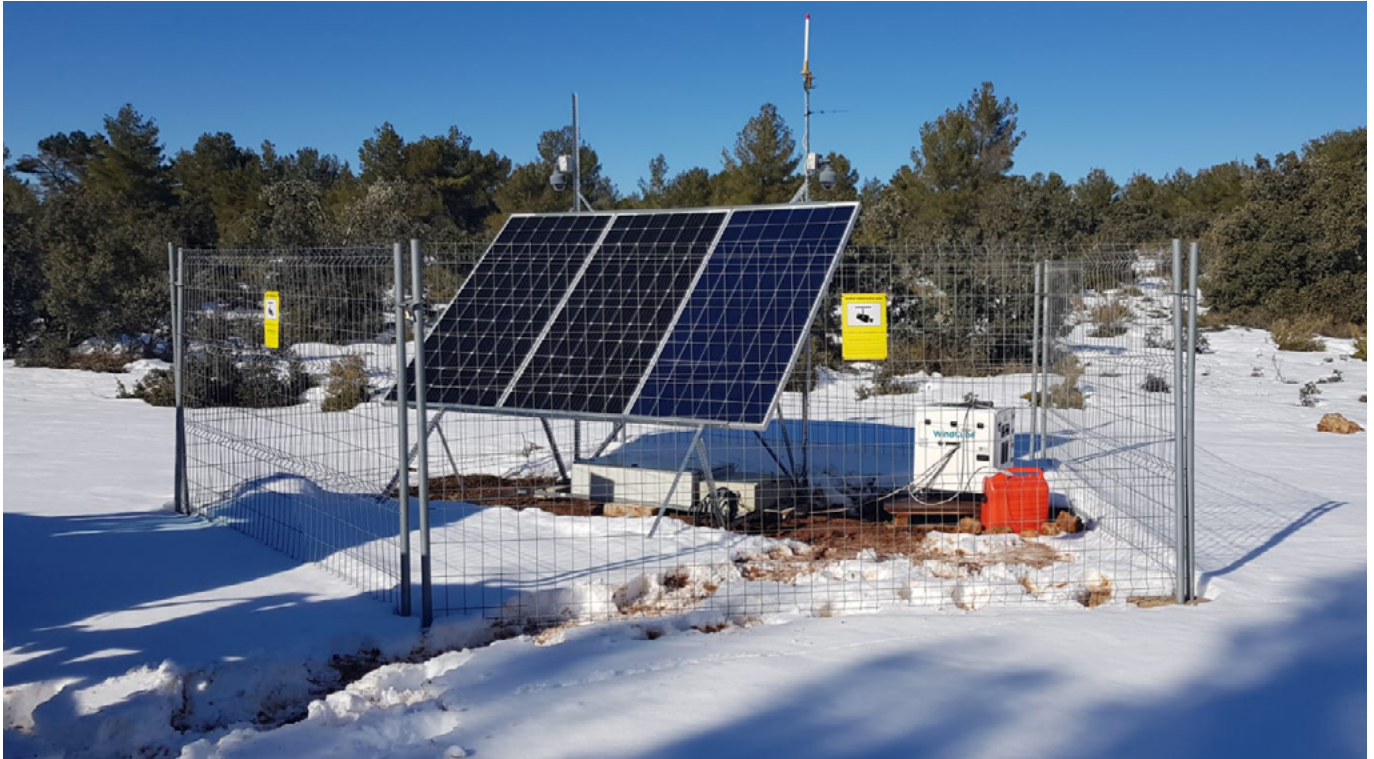
Figure 14: WindCube deployment in cold weather conditions — WindCube after a storm in Spain. Courtesy of Barlovento Recursos Naturales.
